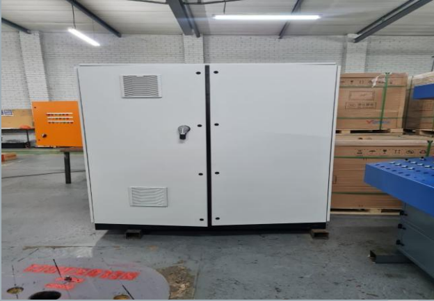
HYDRAULIC TEST CONTROL CONSOLE
