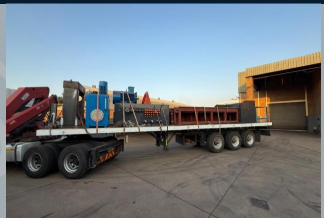
EQUIPMENT PREPARED FOR PROJECT MOBILISATION
